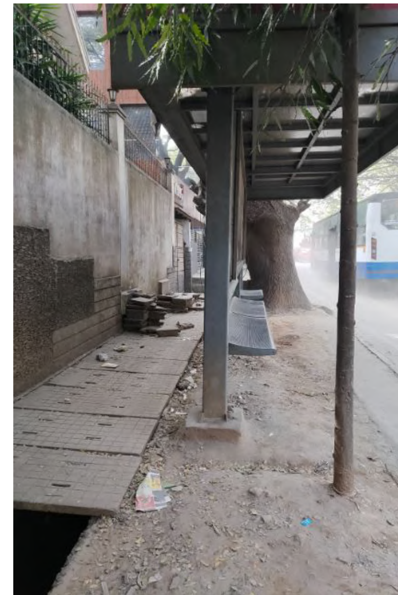
Koramangala water tank bus stop (towards Koramangala) - broken footpath and open drain.
