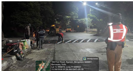
Image: Speed hump executed towards Indiranagar by BBMP TEC.
