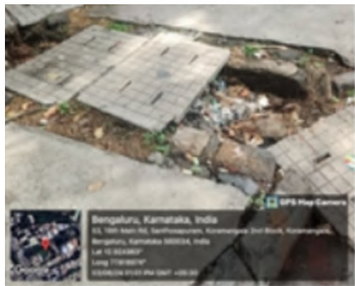
Image: Clogged shoulder drains block the free flow of stormwater.
