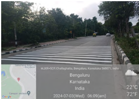
Image: Rumble Strips laid by BBMP TEC.
