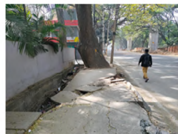
Broken slabs, pavers and open drains in Koramangala
