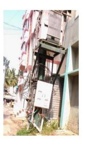
In residential areas, particularly for the power supply to apartments, the existing overhead structures and transformers to be replaced with cubicle type Compact Substations or RMU cum Transformer Units which enable "loop in – loop out" cabling, without any exposed live parts.
